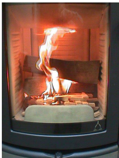
Figure 5: Close the Primary Air
