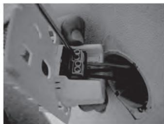
5/ Fasten the support in the standard recessed box ( $\varnothing$  60mm, depth = 40mm).
